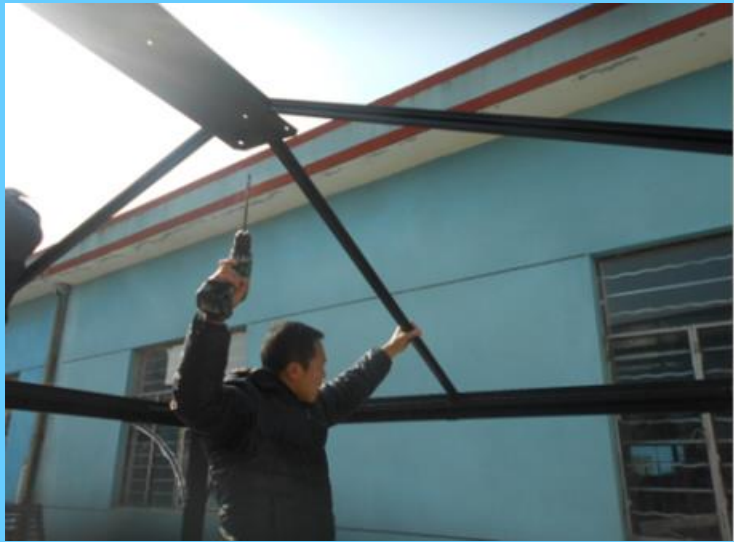
fix the two central ribs
