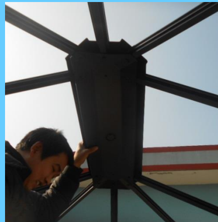
Fix the 4 corner ribs
