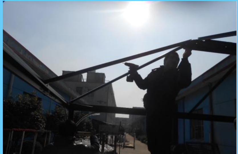
Fix the 4 corner ribs
